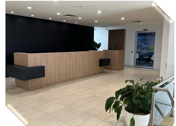
Design & construct fitout of custom workstations, joinery, storage and reception area.
